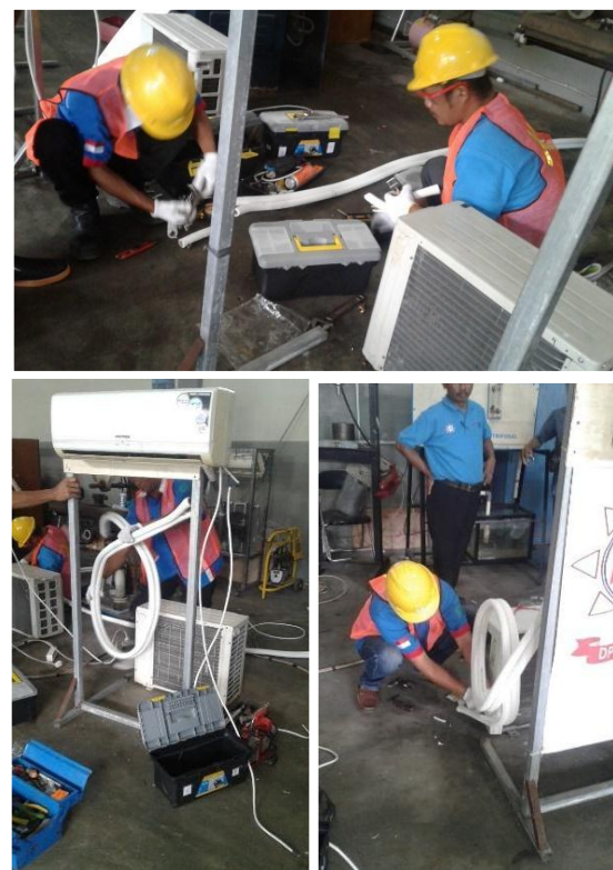
Figure 3. Socialization of SOPs and practice of AC installation, maintenance, and repair.
